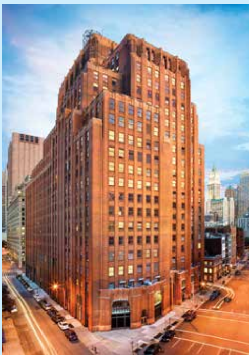
Designated a historic landmark in 1992 by the New York City Landmarks Preservation Commission, the iconic 60 Hudson Street boasts an Art Deco exterior and Guavastino tile ceiling in the main lobby.
