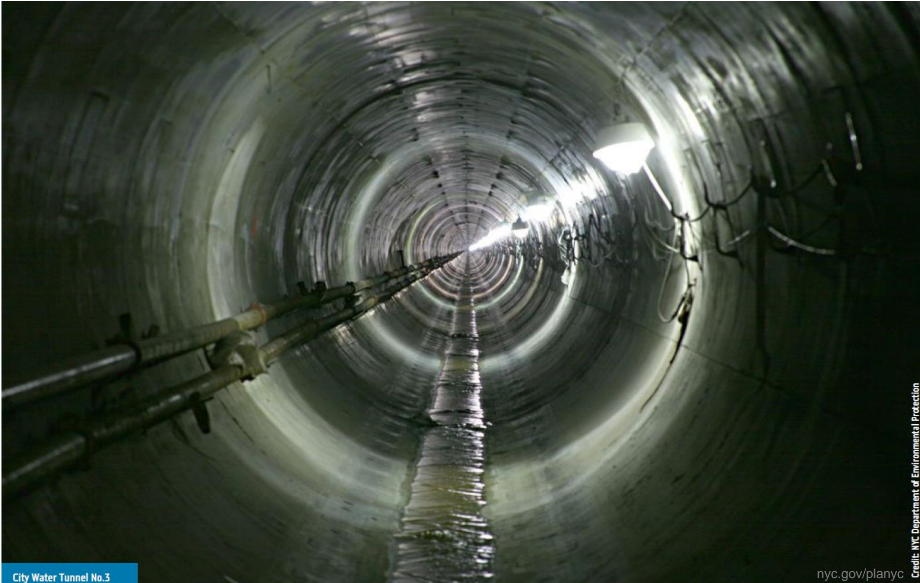
City Water Tunnel No.3
